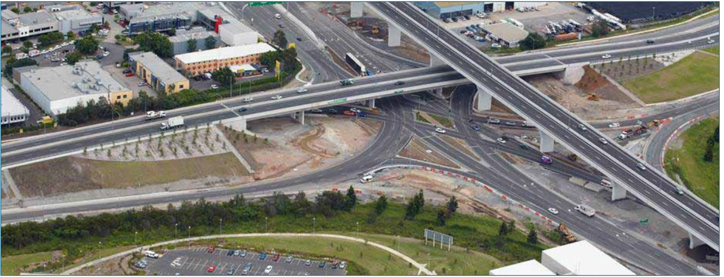
Airport Roundabout Upgrade Project – looking North West
