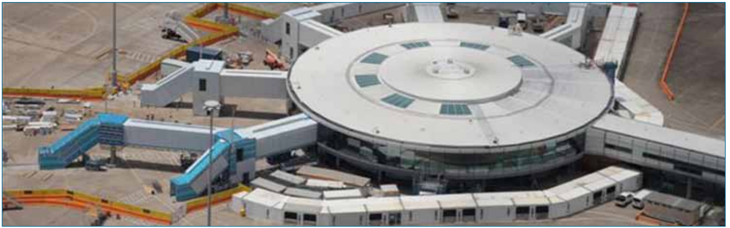
Common User Satellite nears completion at Domestic Terminal
