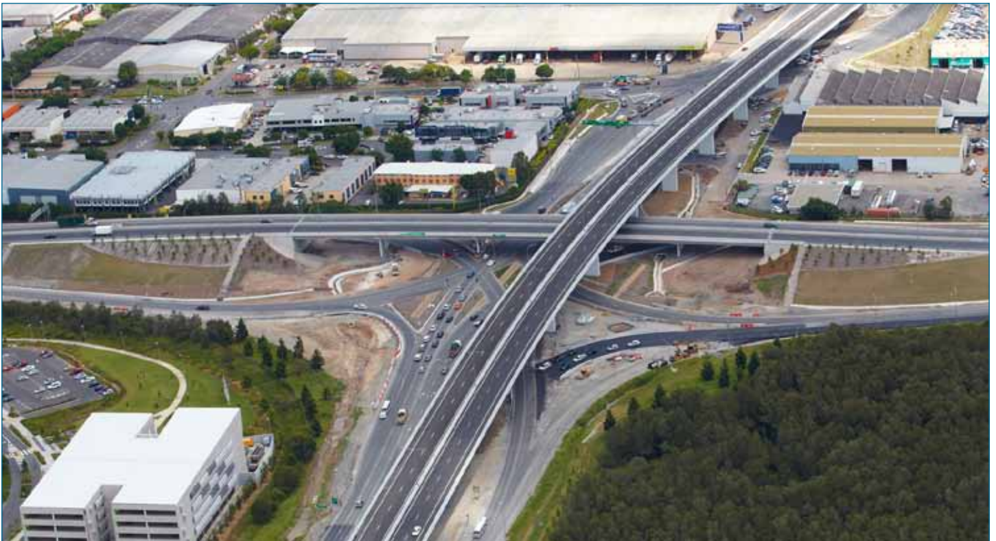
Airport Roundabout Upgrade Project (Late February 2011) – looking North West
