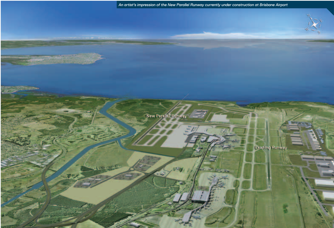
An artist's impression of the New Parallel Runway currently under construction at Brisbane Airport
