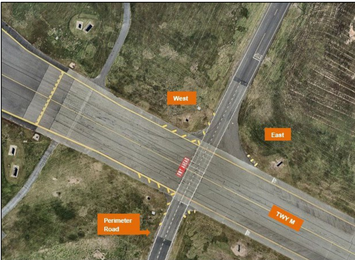
Figure 49 Taxiway Mike / Perimeter Rd
