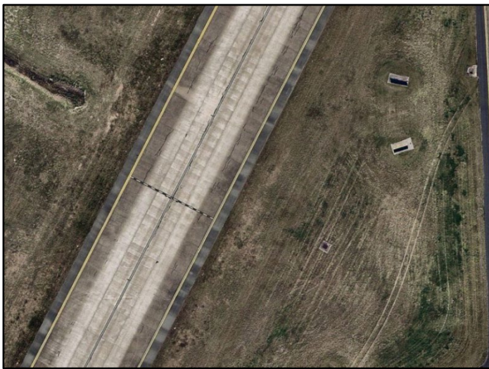
Figure 62 Intermediate Holding Point
