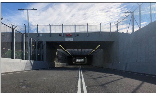
Figure 1 Dryandra Road Underpass Height Restriction
