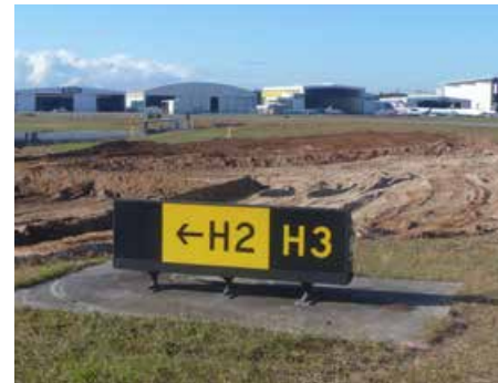
$25m Hotel Taxiway Upgrade
