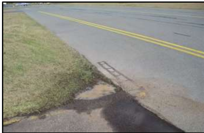
Figure 27 Example of leaving paved areas resulting in mud, grass gravel onto taxiway
