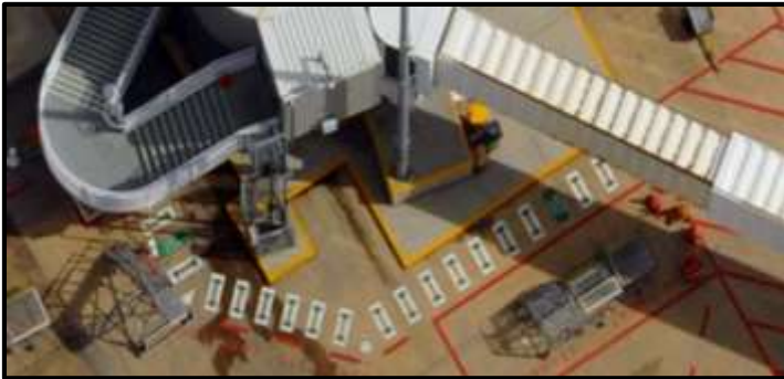
Figure 6 Pedestrian walkway and eye wash station
