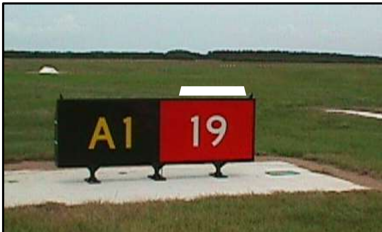
Figure 50 Runway Designation Sign
