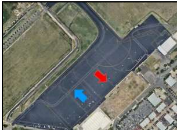
Figure 33 Perimeter Road (Blue Arrow), Aircraft stand (Red Arrow)
