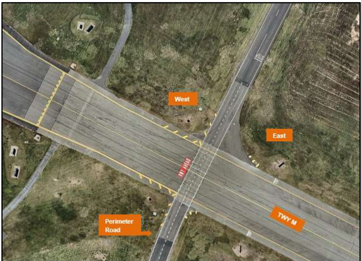
Figure 40 – Taxiway Mike / Perimeter Rd
