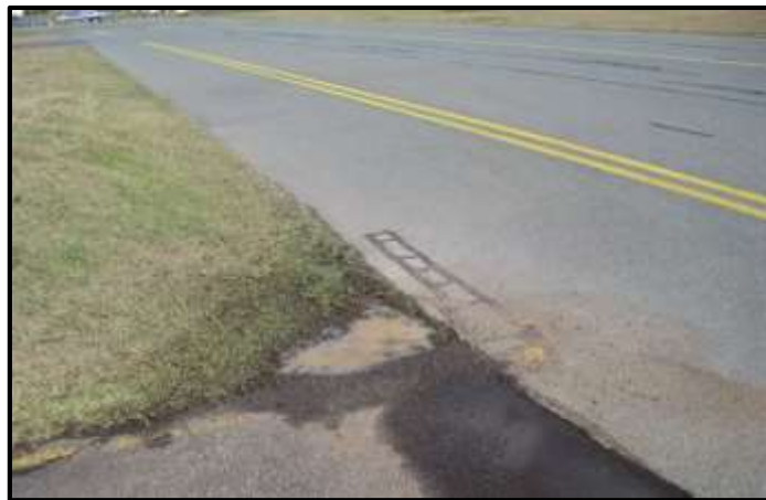
Figure 27 Example of leaving paved areas resulting in mud, grass gravel onto taxiway
