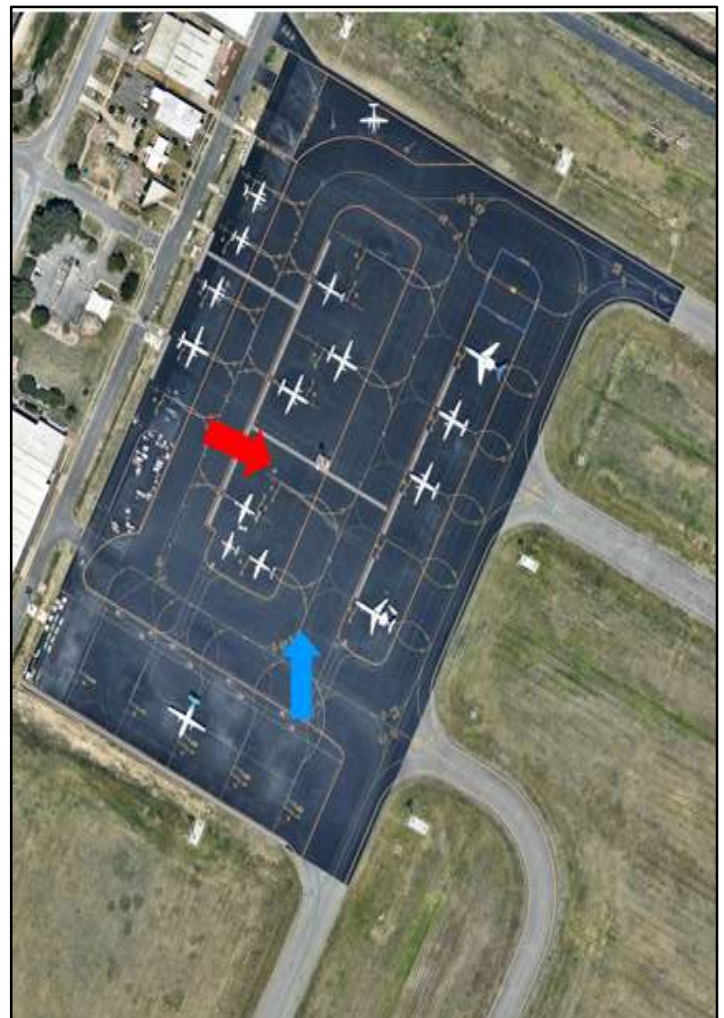
Figure 35 Apron Taxi Lane (Blue Arrow) Aircraft Stand (Red Arrow)
