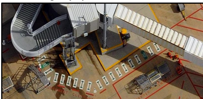
Figure 6 Pedestrian walkway and eye wash station
