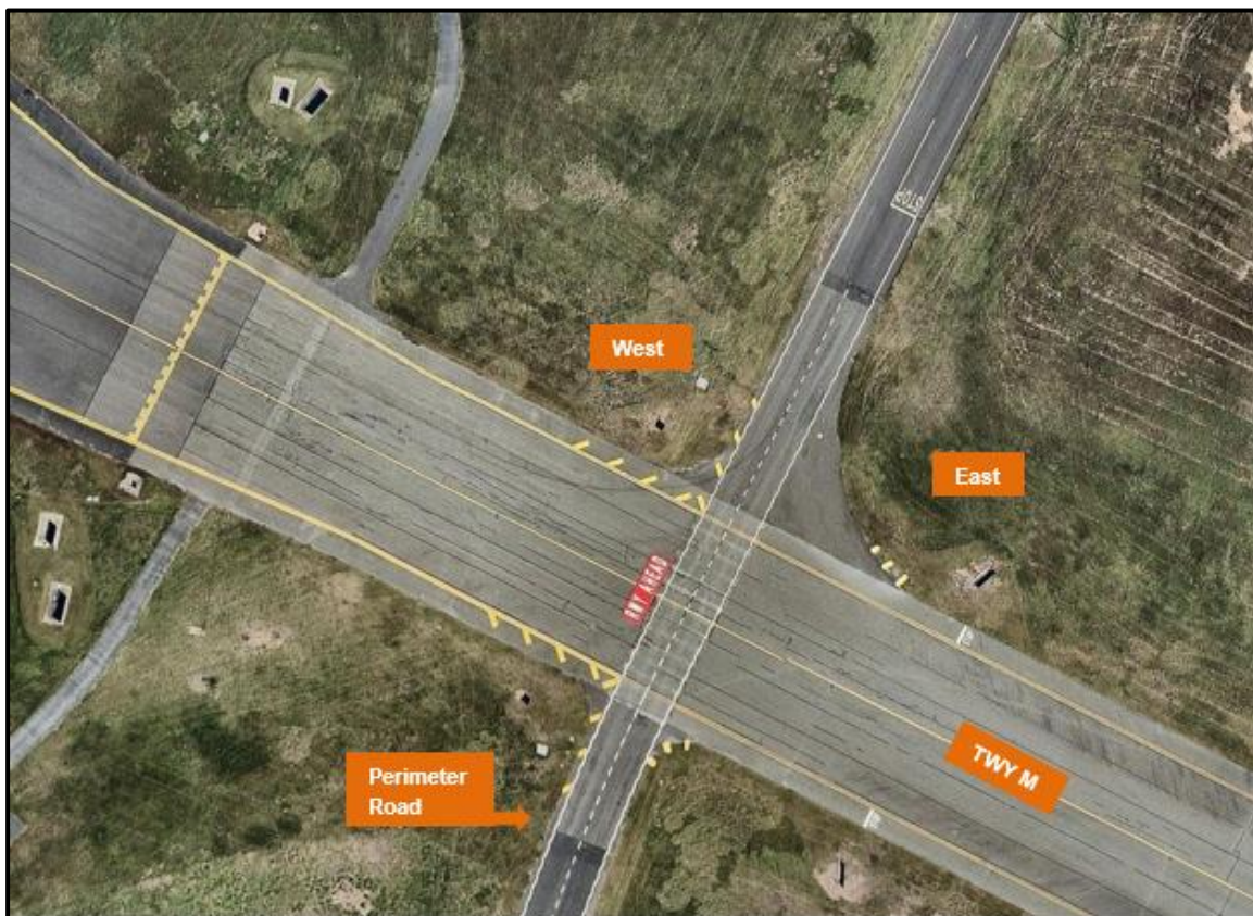
Figure 40 – Taxiway Mike / Perimeter Rd
