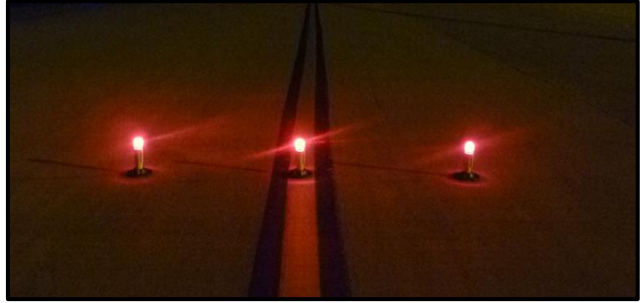
Figure 48 Red Steady lights replace U/S Cones at night
